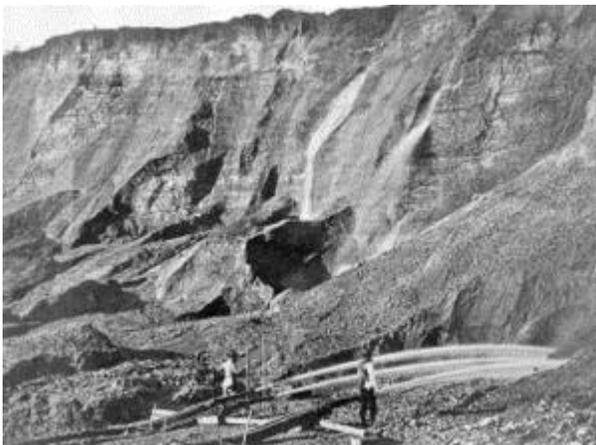
Gold miners excavate a gold-bearing bluff with jets of water at a placer mine in Dutch Flat, California, sometime between 1857 and 1870.
